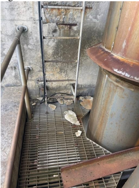
Figure 1: Image showing spalled concrete on the steel walkway
