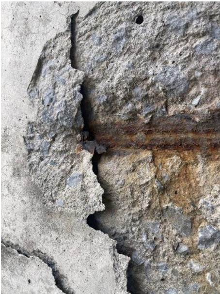
Figure 2: Image shows loose concrete
