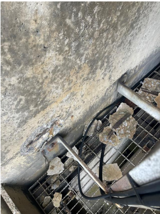
Figure 3: Image shows spalled concrete at the access ladder connection
