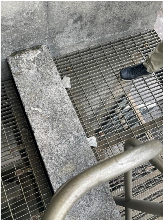
Figure 4: Image showing piece of fallen concrete and a crack in concrete beam
